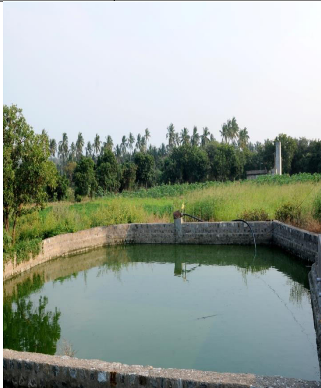
Bore Well, Open Well and Water Recharge
